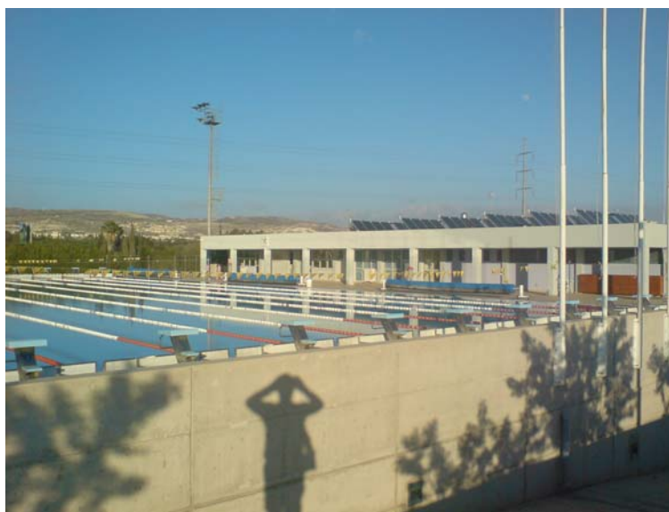
Figure 8: Solar collectors next to the swimming pool
