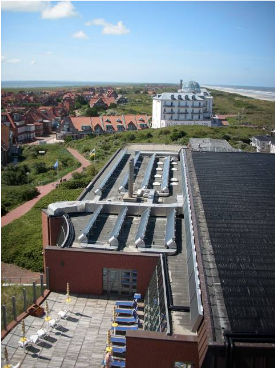
Figure 7: Combination of air collectors and unglazed absorbers
