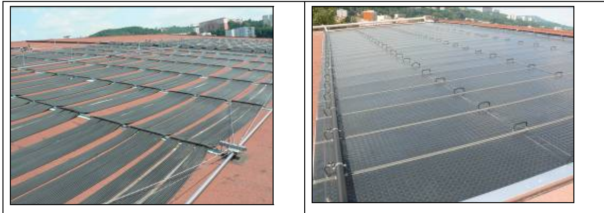
Figure 8: Swimming pool of Vaise in Lyon, France (Source: ALE)
